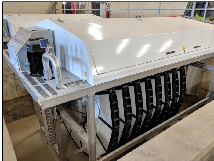
Figure 9 – Inside-Out Cloth Disk Filter Schematic
