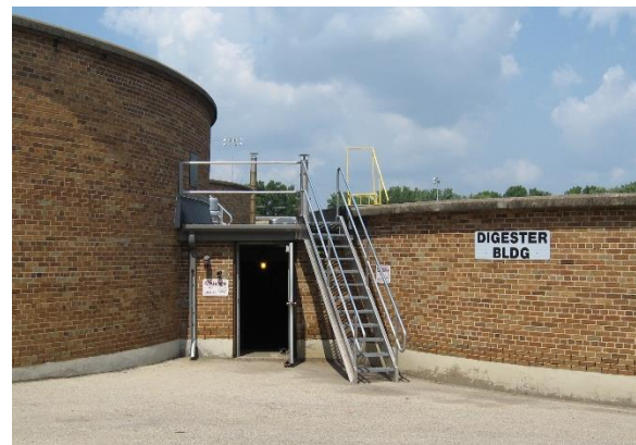
Figure 14 - Anaerobic Digester Complex
