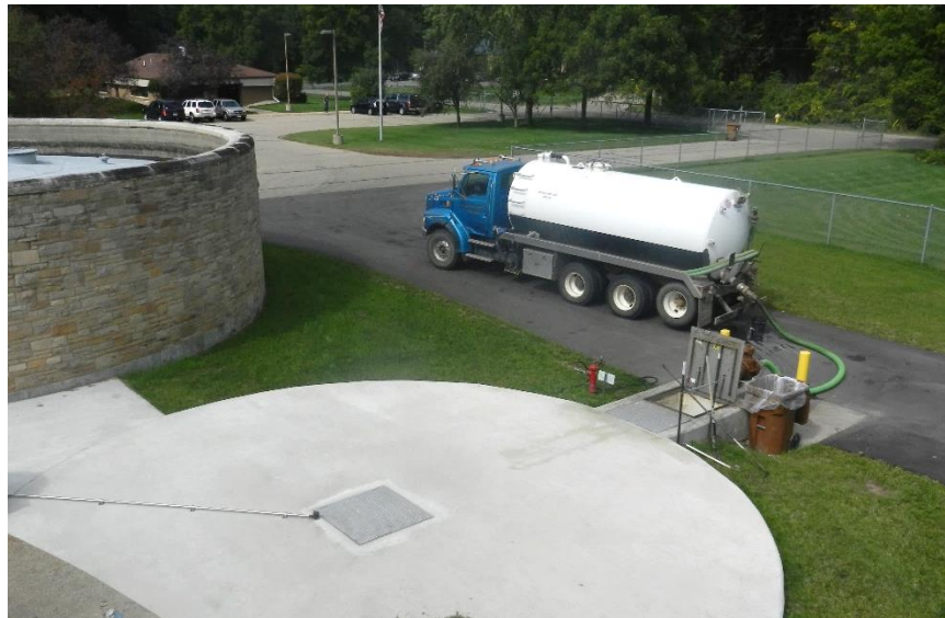
Figure 3 – High Strength Waste Receiving
