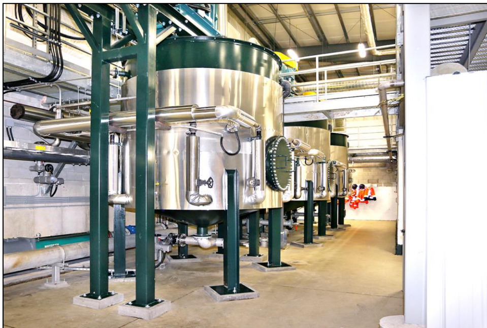
Figure 22 – Thermal Hydrolysis Reactor Example
