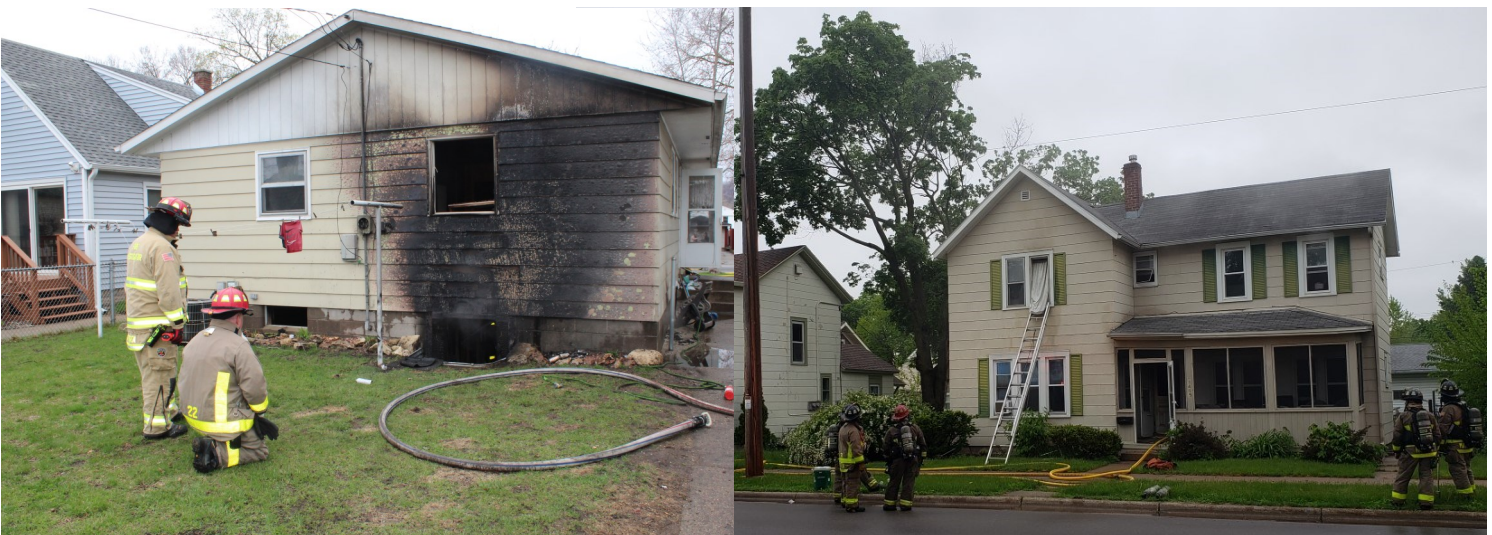
2022 Investigated Fire Incidents
