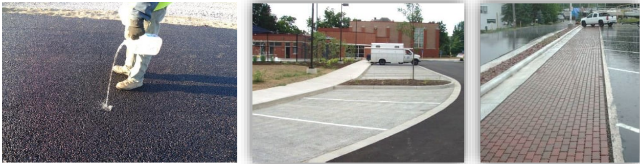
Figure 4.03-5 Permeable Pavement Options
